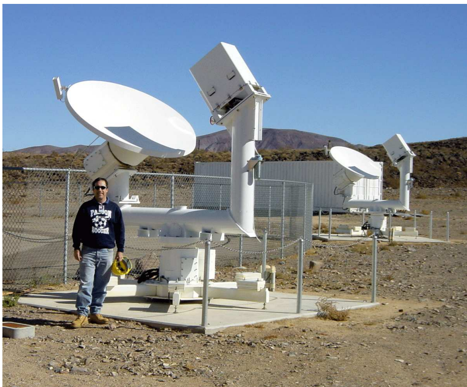
Figure 11: Two water-vapor-radiometer-based Advanced Media Calibration units located near DSS 25, shown here in November 2001. These are used to calibrate tropospheric phase scintillation for the Cassini Gravitational Wave Experiment and other Cassini precision Doppler tracking observations. (Mark Gatti, project manager for the Cassini Radio Science ground system upgrades, is in the foreground.)
