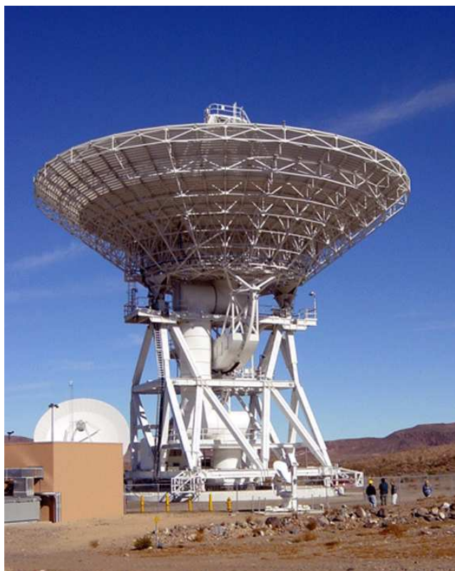
Figure 3: DSS 25, a 34-m beam-waveguide antenna, shown here in the stowed position. DSS 25 is one antenna in the NASA/JPL Goldstone Deep Space Communications Complex near Barstow, CA, U.S.A. It has special instrumentation (Ka-band up- and downlink and advanced tropospheric calibration capability) which enable particularly good quality Doppler observations.
